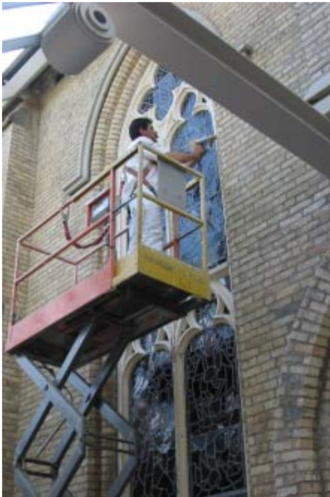
(Above) Several repair and maintenance jobs were done while the sanctuary was empty for the summer. Hugh Godau of Paramount Painters was able to scrape and paint the frames on the stained glass windows facing the atrium without disturbing anyone.
